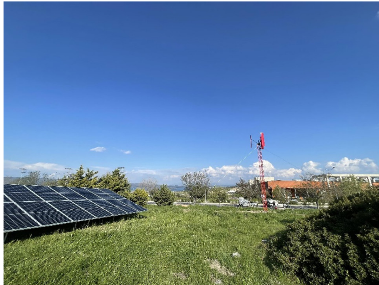
Figure 4: The vertical axis wind turbine used in the project
